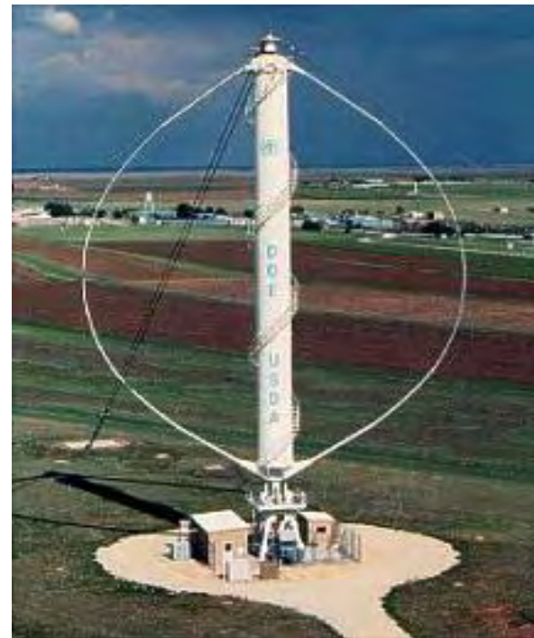
Sandia 34 m Darrieus Sandia National Labs
